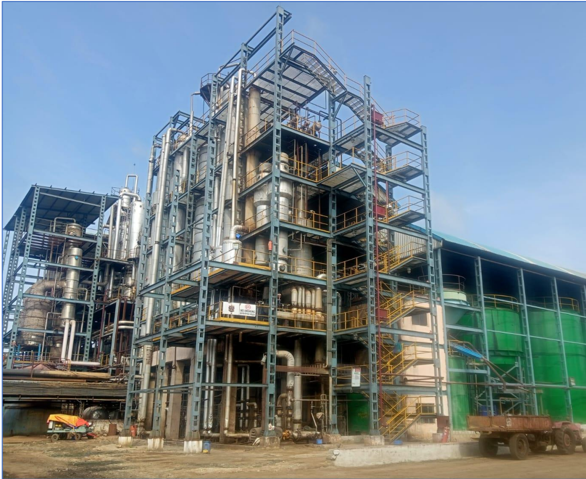
Photograph showing the project site
